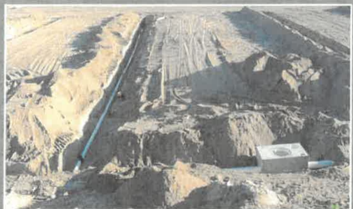
Example Infiltration Treatment Basin Under
