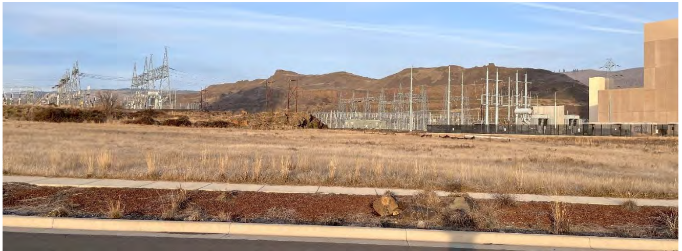
Figure 5: Port of The Dalles Property Lot 25
